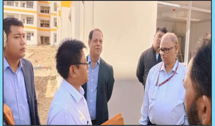
SITE PROGRESS VISIT OF MSME TECHNOLOGY CENTRE IMPHAL BY THE THEN SECRETARY, MINISTRY OF MSME, B B SWAIN AT THE NEWLY CONSTRUCTED BUILDINGS ALONG WITH THE OFFICIALS
